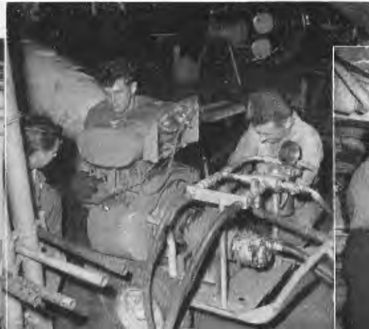
Mending ground equipment
