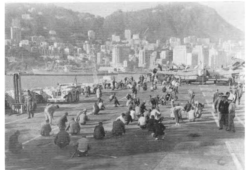
Chinese contract labour chipping the Flight Deck
