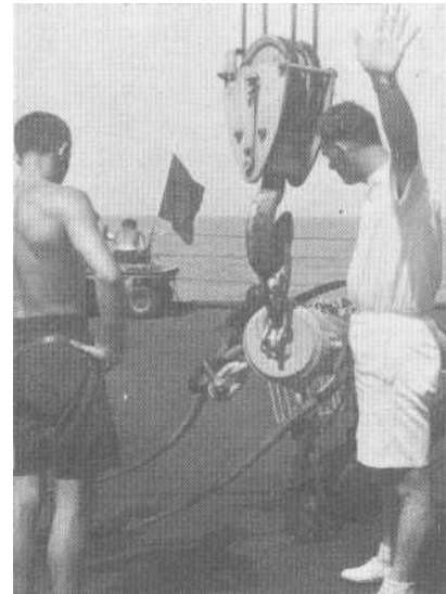
RAS Solids. Rigging the
