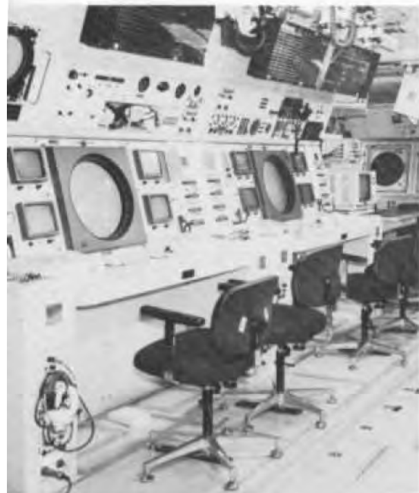
CACS consoles in the Ops Room
