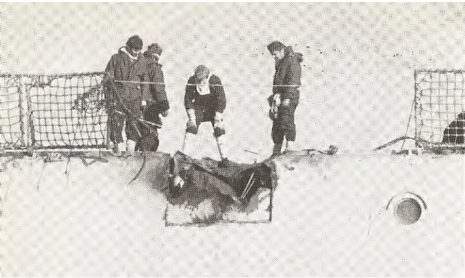
Bomb damage to the flight deck. A fully primed mortar bomb on the deck exploded having been hit during an Argentine Air Raid.
