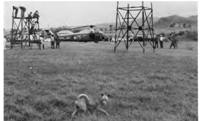
Sections 4 and 5 are being prepared for practice lift
