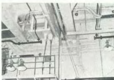
Fire precautions are of paramount importance. In the spacious hangar fire curtains are fitted - shown (right) in the stowed position outside the hangar control room.
