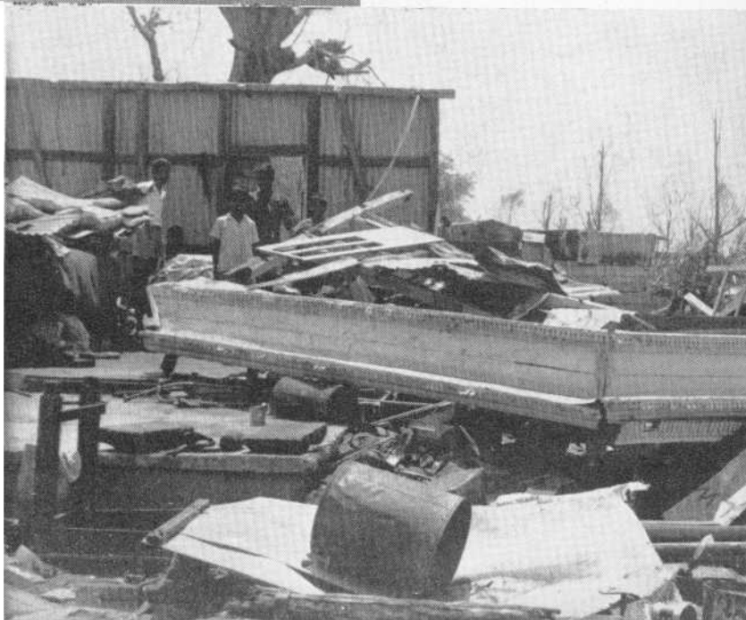
The day the roof fell in
