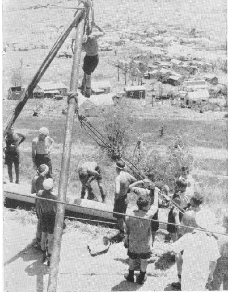
Essential services maintained - All in a day's work
