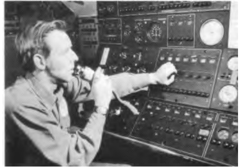
Systems control console in the Control Room.
