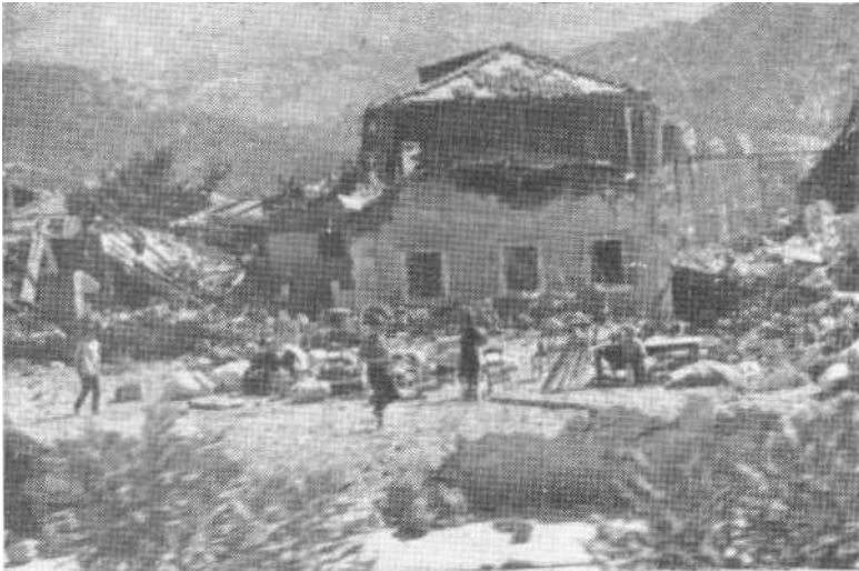
Some of the damage at Argostoli after the Earthquake
