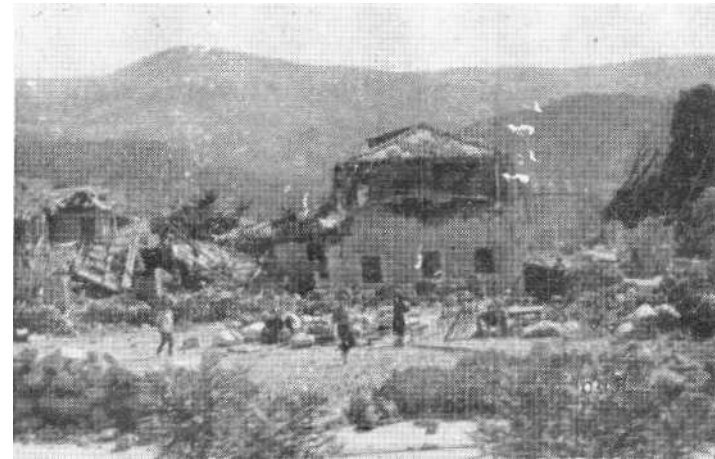
Our photo shows the extent of the damage.
