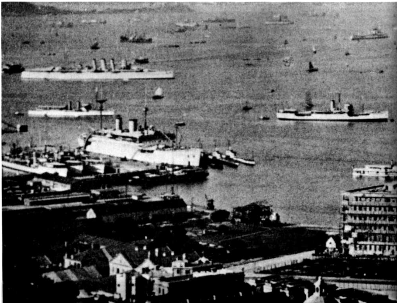
The China Fleet Club still in scaffolding - 51 years ago in 1933!
