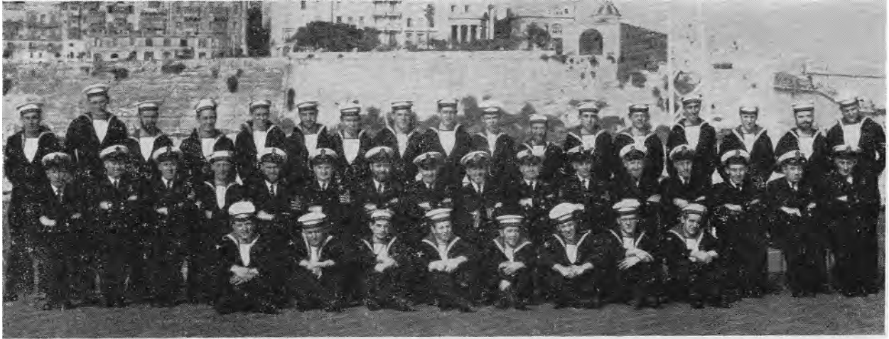
ENGINE ROOM DEPARTMENT - 'X' UNIT DIVISION
