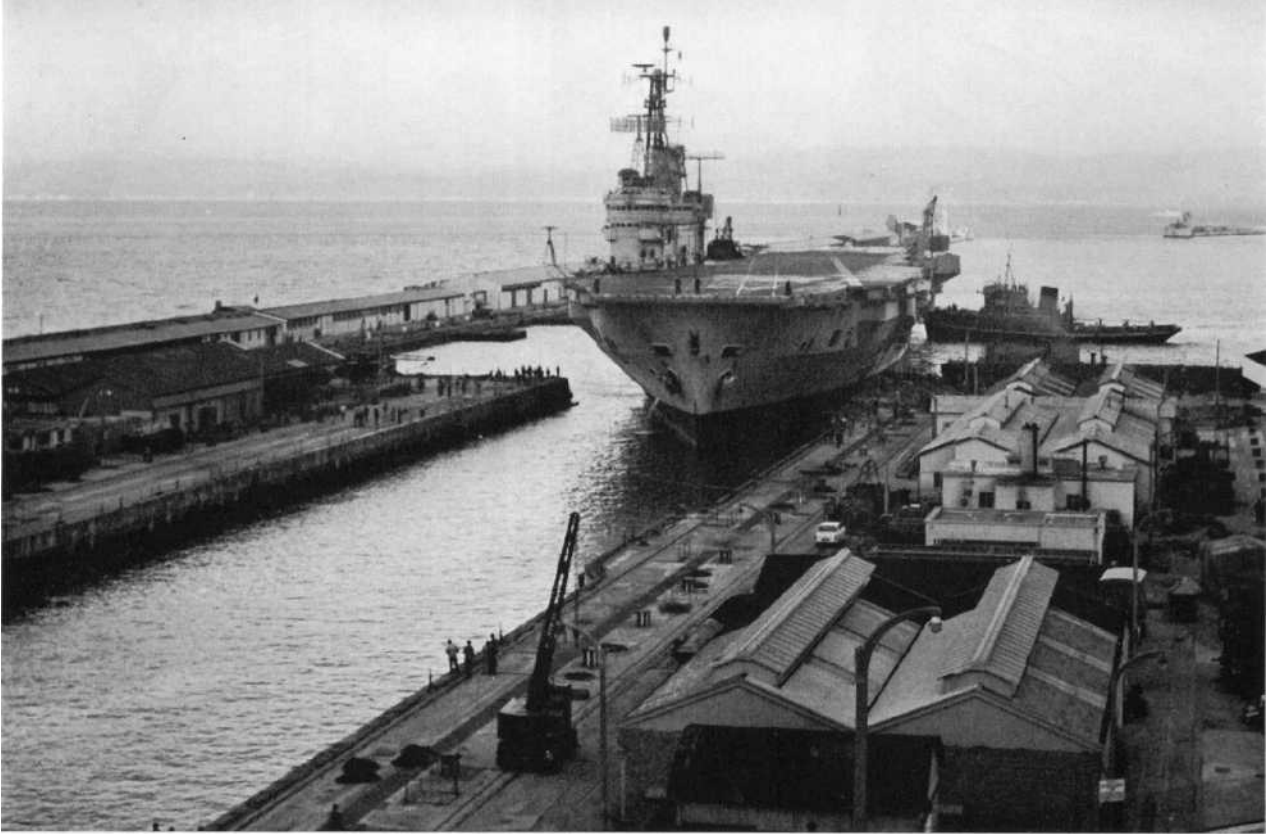
ENTERING NO. 1 DOCK
