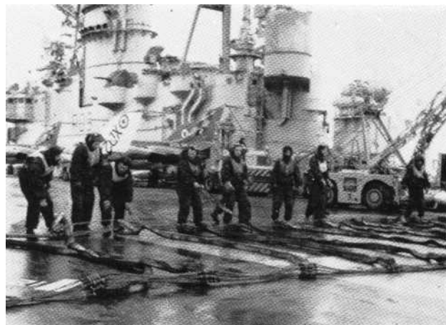
Rigging the barrier
