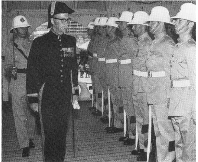
Guard Inspection - Consul General, Capetown
