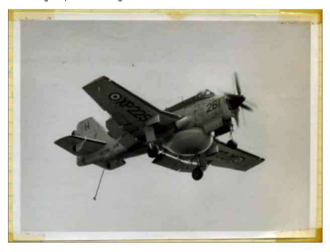
AEW Mk 3 Gannet (XP225) flying round on its last circuit. Note: Arrester-hook, Undercarriage and Flaps down
